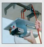
The hoist tool makes it possible for only one person to install a PROTECT Fog Cannon. And it is safer - you are taking care of your back and do not fall down the ladder with a lot of kilos in your hands.
