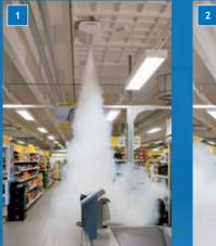
A burglar breaks through a window and triggers a sensor. Both the alarm system and the fog cannon are activated and the room is filled with a white, dense, dry fog, so the burglar can't even see his hand in front of his face! He does the only thing he can - turns around and runs out the same way he came in.
